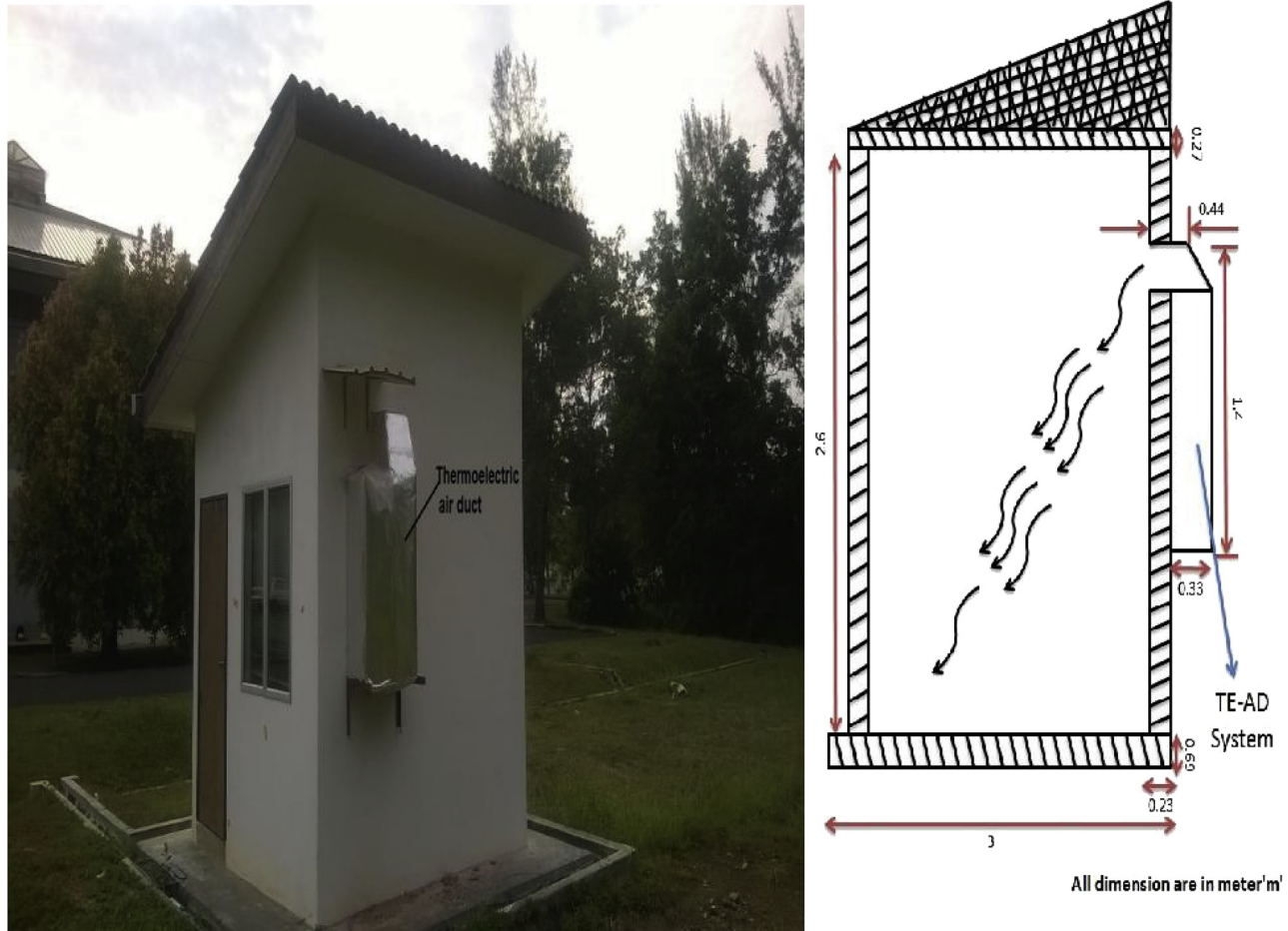
Fig. 1. Test room equipped with TE-AD system.
