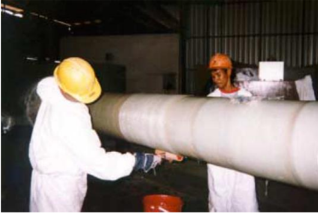
Figure 4. Composite combined corrosion and fire protection applied to a platform jacket leg.
