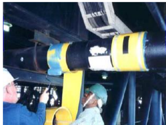
Figure 1. Offshore application of a 'Clockspring' repair to an externally corroded pipe
