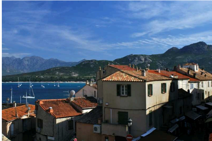
Figures 1. Roofs that are exposed to direct sunlight, taken from [3]
