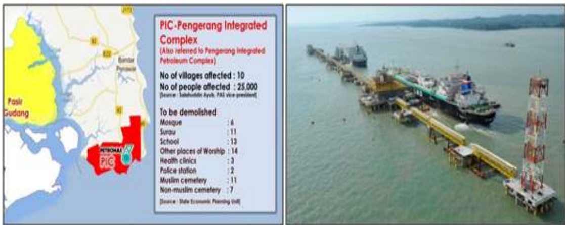
[ Pengerang Integrated Complex, Johor주(좌)와 LEKAS, re-gasification facilities, Malacca(우) ]
